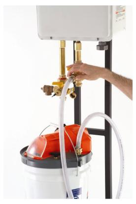
2. Connect the return hose to an access valve
