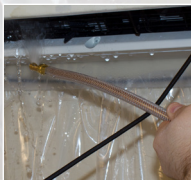
Clean fan blades and blower wheel
