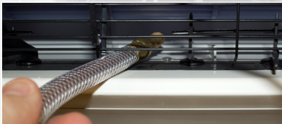
Clean inside the system
