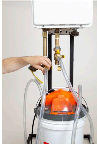
Connect the return hose to an access valve.
