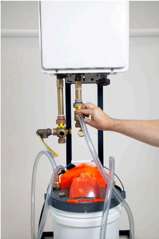
Connect the outlet hose to an access valve.
